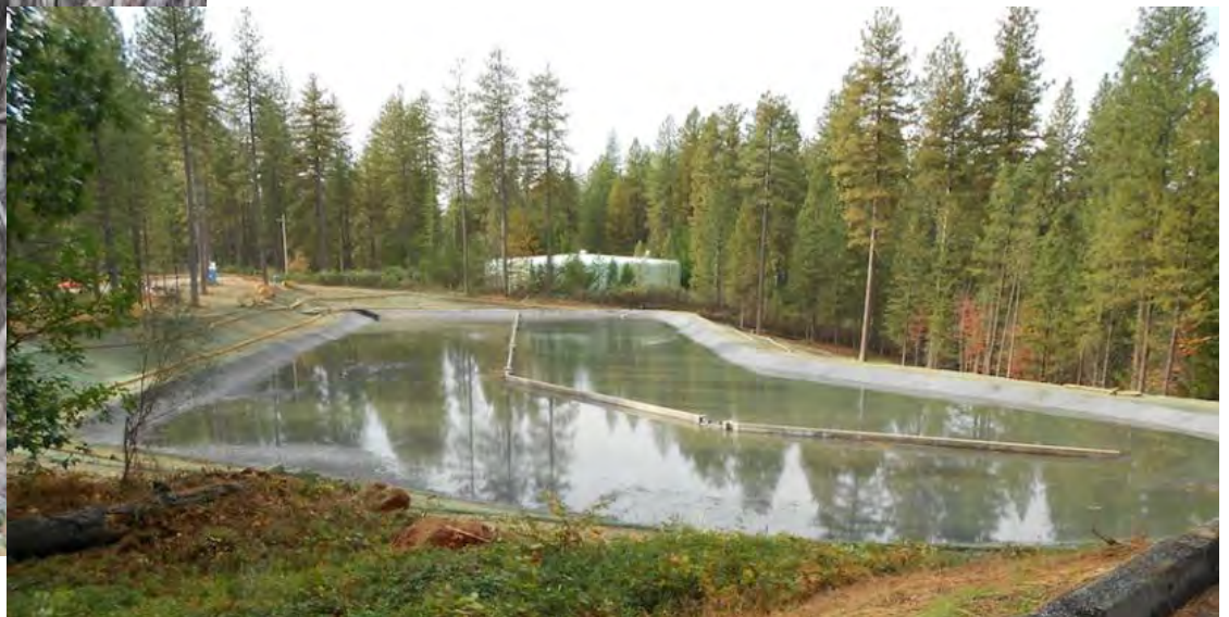
Anoxic limestone treatment in finishing pond
