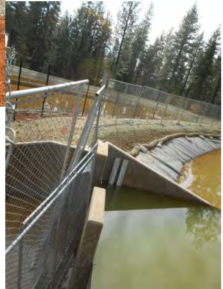
2 - Outfall from Settling Pond to Wetland No.1
